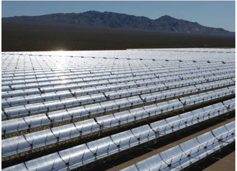
Photograph of Nevada Solar One provided courtesy of Acciona
